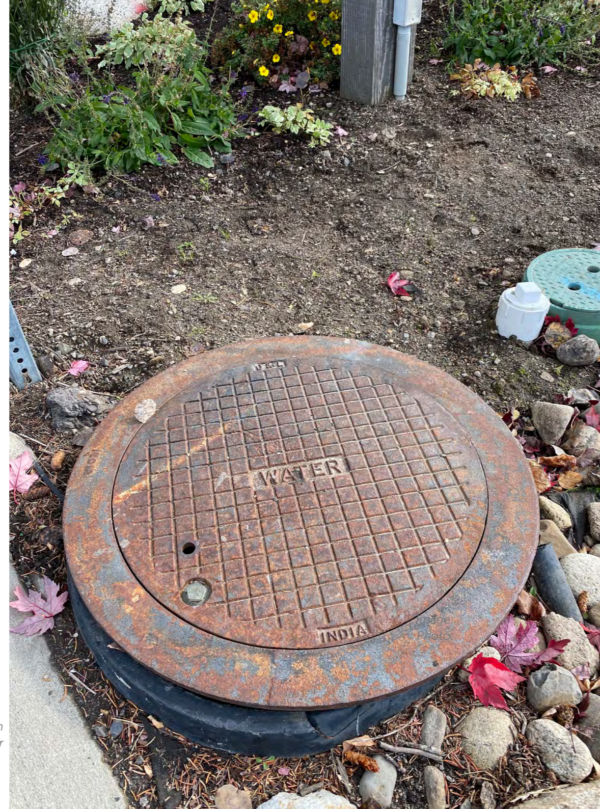
Utility cover near public restroom Photo: Amy Westover
