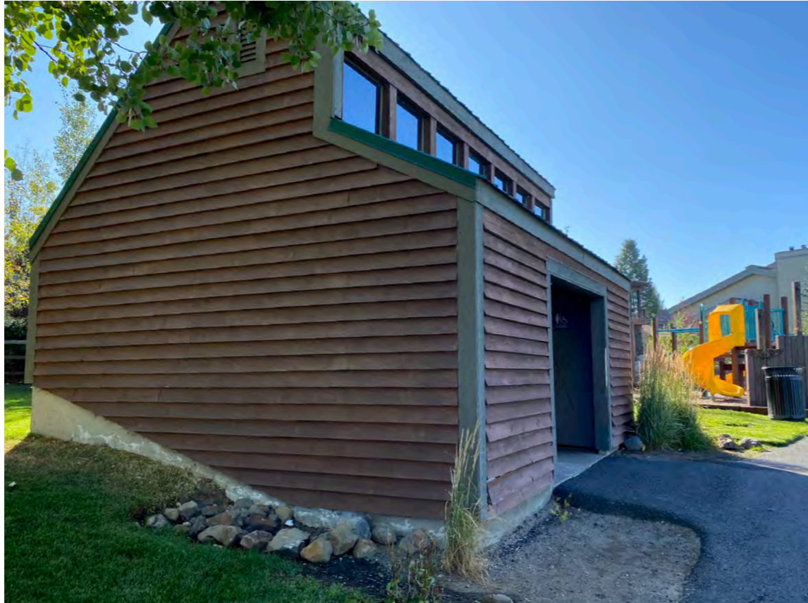
Restroom at Brown Park Photo: Amy Westover
