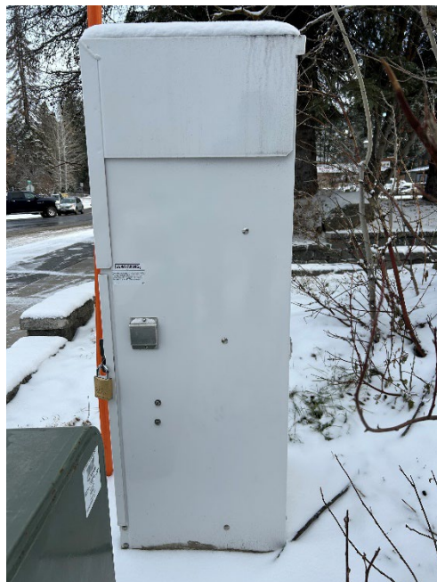
Photo of a streetlight control box to receive artwork vinyl wrap.
