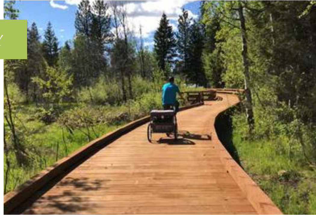
Wooley Boardwalk over protected wetlands. Photo: City of McCall.
