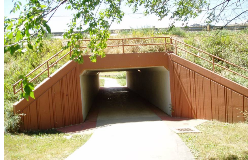
Figure 40: Grade separated crossing, Boulder
