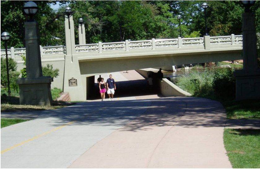
Figure 39: Grade separated crossing, Boulder
