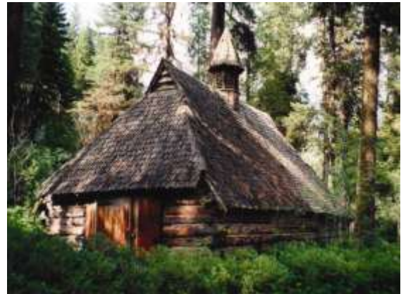
The Sylvan Beach Ice House built ca. 1932 supplied ice to the resorts cabins until 1943. Notice the shake roof and tall octagonal cupola.
